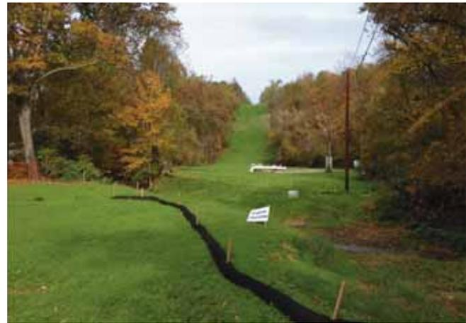
**Figure 4.** EOT pipeline project in Alleghany County, Pennsylvania, on 10/15 after EarthGuard Fiber Matrix was applied.
