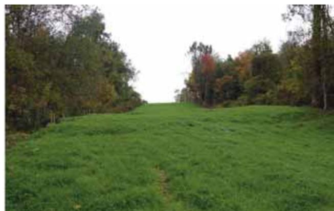
Figure 2. EQT pipeline project in Allegheny County, Pennsylvania, on 10/15 after EarthGuard Fiber Matrix was applied.
